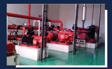
The Hydrant System comprises of AC motor driven pump sets with all required accessories including valves, instrumentation and controls etc. Complete in all respects. An automatic hydrant system is furnished covering the areas completely from independent. Pipe work from the fire water pump set. The hydrant pipe work is remaining pressurized through the proposed jockey pump taking care of any leakages in the system pipe lines, valves and fittings.
